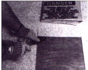
working the scraper beneath the tile and exerting both a forward pressure and a twisting action on the blade to promote release of the tile from the adhesive and the floor.
